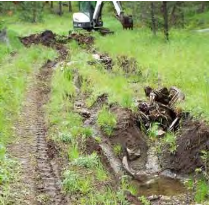
Figure 2 Excavator starting to re-direct water flow
