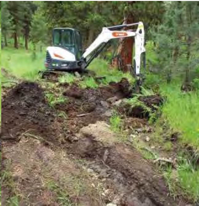
Figure 3 Cleaning culvert and berming road
