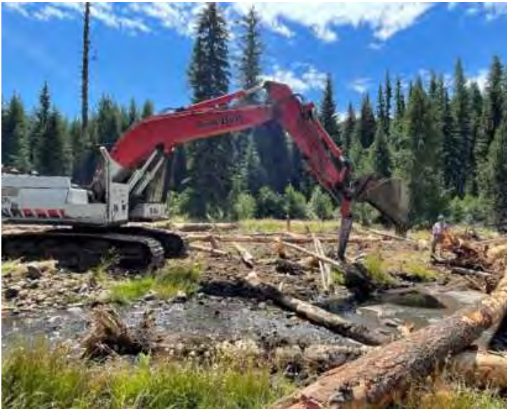
Excavator placing large wood on the floodplain
